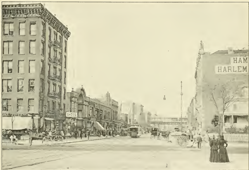
ONE HUNDRED AND TWENTY-FIFTH STREET, LOOKING WEST FROM SEVENTH AVENUE.
